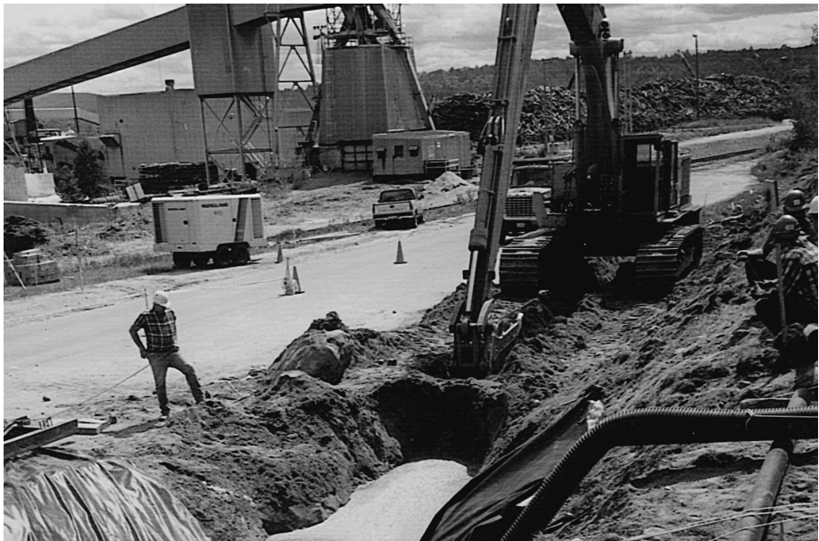
Fig. 4. Biopolymer slurry trench construction.
